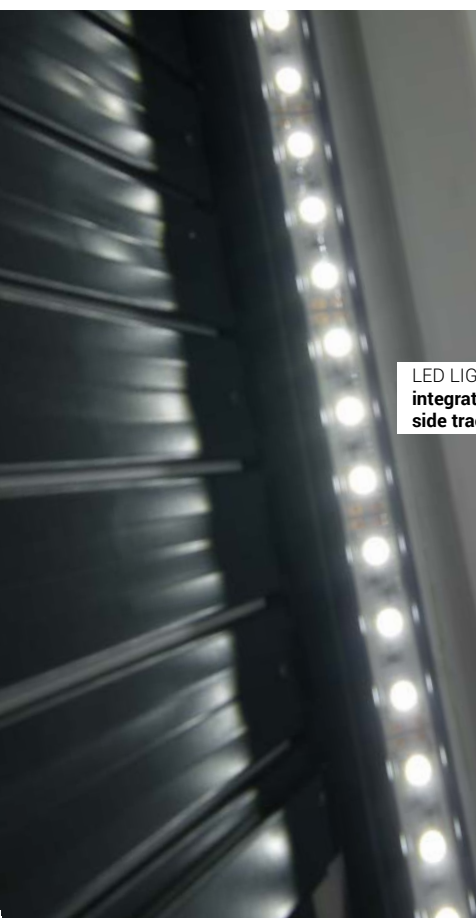
OUTSIDE AREA LIGHTING integrated in a drip channel
